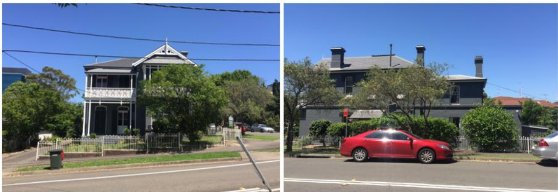
Figure 14 – View of 53 Sorrell St (left) and side view from Harold St, part of subject site and heritage item. Source: Heritage21
