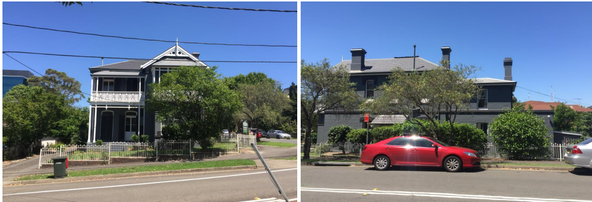
Figure 2 – View of 53 Sorrell Street (left) and side view from Harold Street, part of subject site and heritage item.
