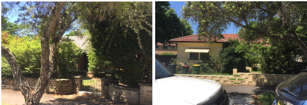
Figure 4 – View of 25 Harold Street (left) and 27 Harold Street (right), part of subject site.
